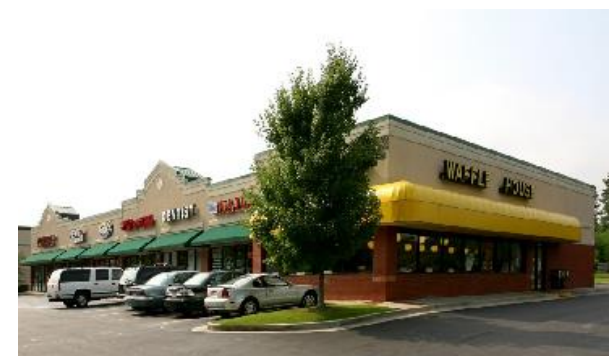
Holcomb Bridge Promenade (11,000 SF)
