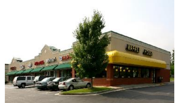
Holcomb Bridge Promenade (11,000 SF)
