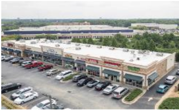
South Point Pavilion (19,219 SF)
